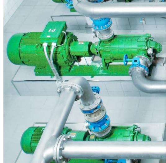
The new ErP (Energy-related Products) Directive requires that – from 1 January 2015, motors with a rated output of 7.5–375 kW must meet IE3 standards (or IE2 standards while being coupled with a variable speed drive).
